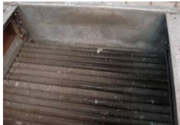
Figure 7b View on top row of finned tubes
